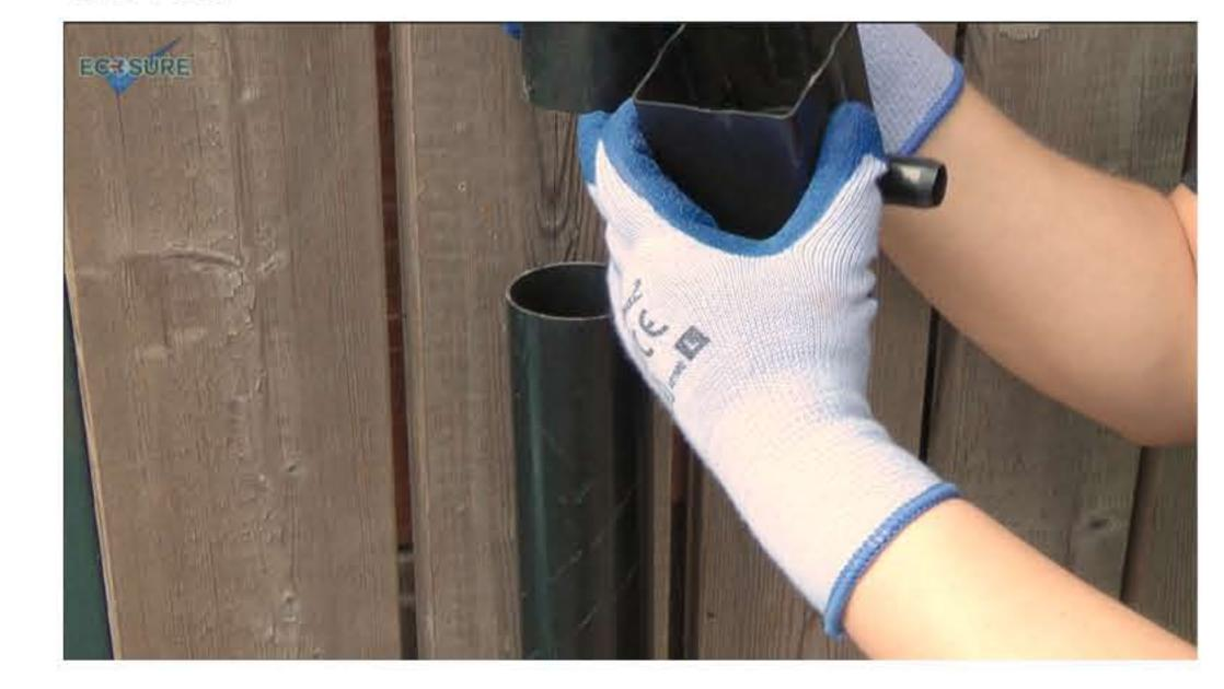
d. Trim the connecting pipe if required, and push one end on to the diverter. Push the other end through the seal fitted onto the tank. Lubricate if necessary.
