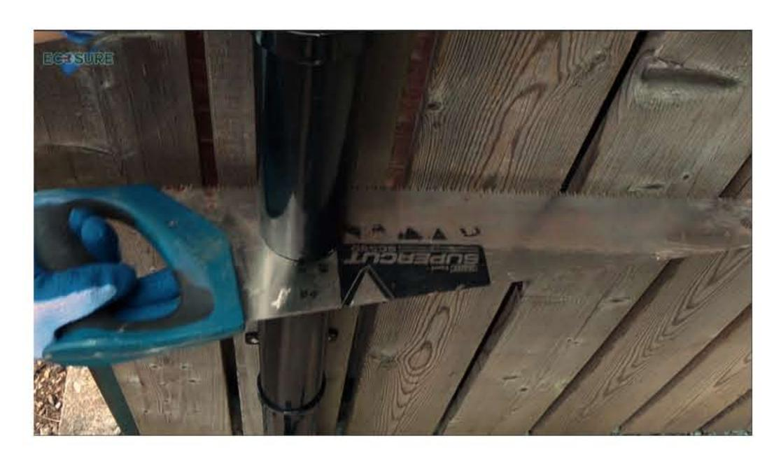
c. Fit the rainwater diverter to the downpipe according to the manufacturer's installation instructions.
